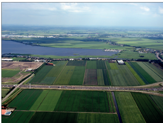
Photo 1.3 (a) Land take by infrastructure (A4 motorway in the polder Haarlemmermeer, near Amsterdam Schiphol Airport, Netherlands)
