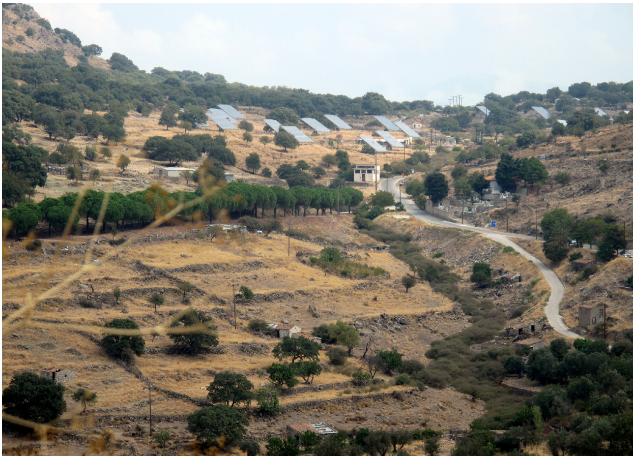
Photo 5.2 Forest encroachment and photovoltaic panels installed on abandoned agricultural terraces (Lesvos, Greece)
