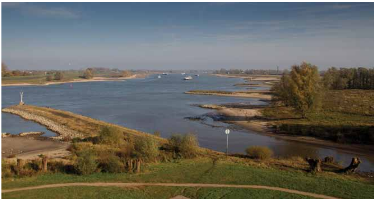
Figure 2.2 Illustration of Room for the River: a widened riverbed increases river discharge capacity
