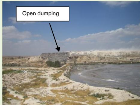
The landfilling method currently practiced involves unloading of solid waste openly, where it is subjected to spreading. Compaction is not applied due to mechanical failure of the compactor and lack of spare parts. Cover material is obtained from within the site area as a result of cells excavation. It consists mainly of sandy soil and it is applied on a daily basis. Thickness of daily cover ranges between 30cm - 50cm.
