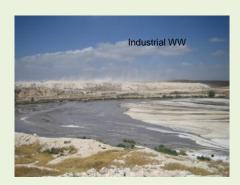
These ponds can be distinguished into two categories: the ones that are situated on southwest side of Al-Ekaider site, are used for disposing olive oil mill wastewater, whereas the remaining ones are used for disposing all other types of industrial wastewater (garment, textile, slaughterhouse, dairy, cement, etc), municipal (untreated) and leachate generated from the solid waste dumpsite
