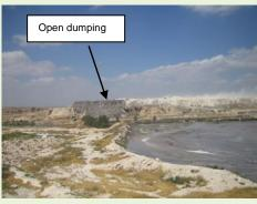
The landfilling method currently practiced involves unloading of solid waste openly, where it is subjected to spreading. Compaction is not applied due to mechanical failure of the compactor and lack of spare parts. Cover material is obtained from within the site area as a result of cells excavation. It consists mainly of sandy soil and it is applied on a daily basis. Thickness of daily cover ranges between 30cm - 50cm.
