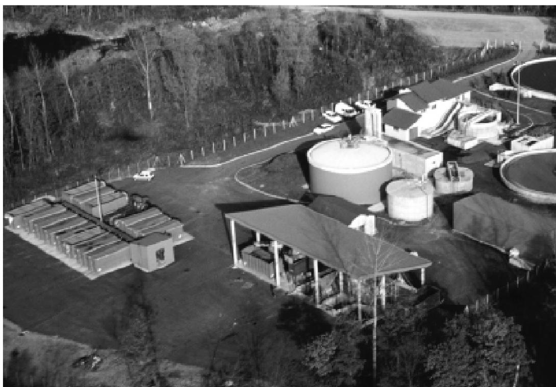
Sludge composting plant of La Roche sur Foron (France): example of an in-vessel composting system.
