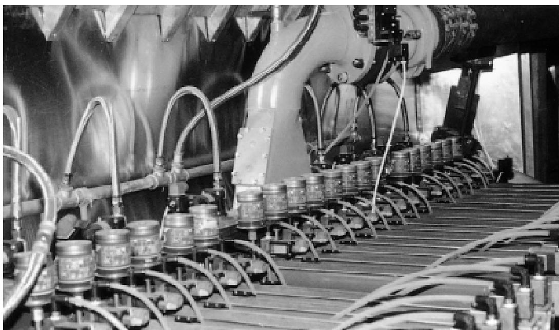
Injectors of sludges used in the incineration plant of Monaco (France)
