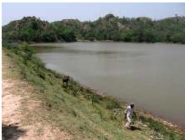
Picture 1: A check dam in Sukhomajri, built to conserve surface water runoff
